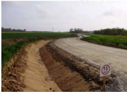
GP - SuDS construction awaiting check dam reinstatement
