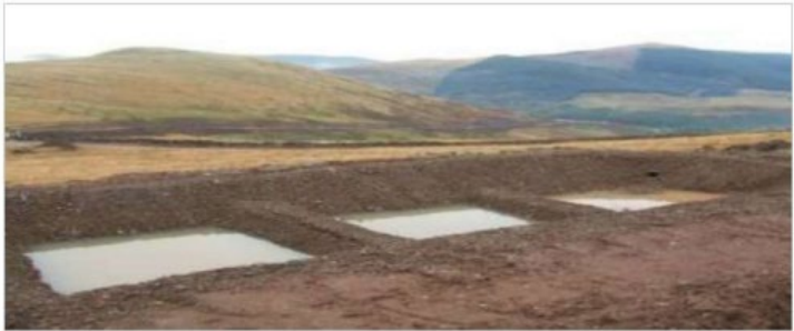
In some locations substantial 'Step' designed settlement lagoons may be required to manage large volumes of contaminated run-off.
