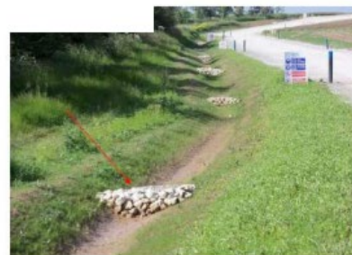
GP - SuDS with check dams installed and maintained and good vegetation from grass seed as per Ecology Plan
